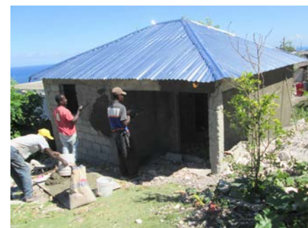
A newly-completed Happy House
